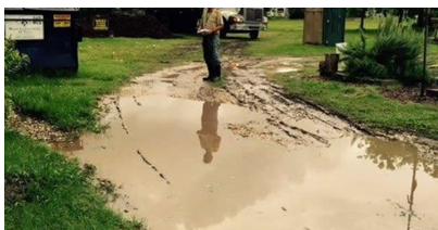
Driveway needs major improvements
