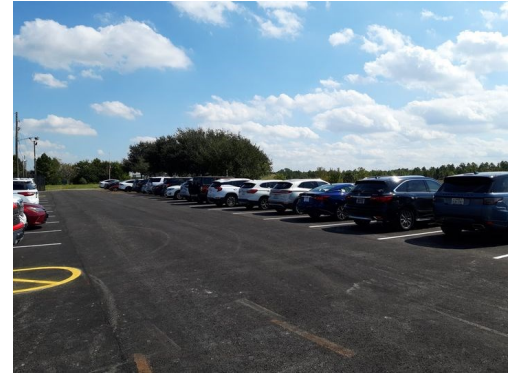
New paved parking lot
