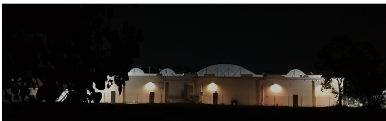
After—New lights installed
