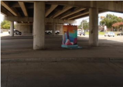
Above: W. Belfort under S. Post Oak after clean-up.
