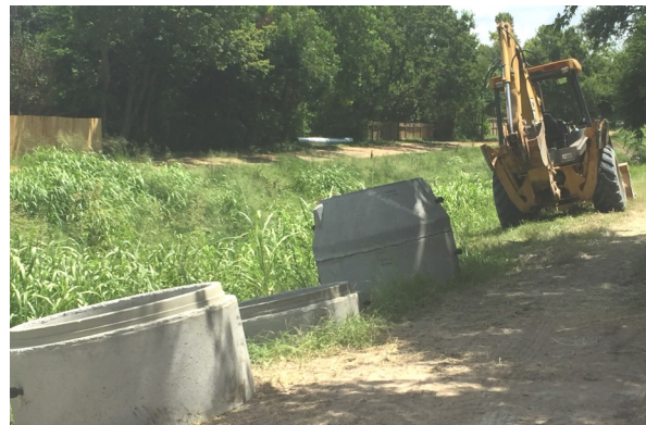
Current repairs to outfall pipes along Willow Waterhole Bayou at Landsdowne
