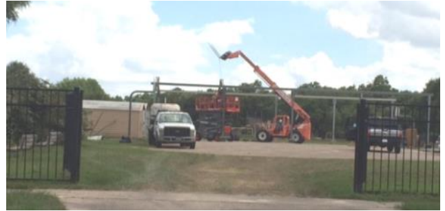
Parker Elementary Demolition Begins with the T-buildings!
