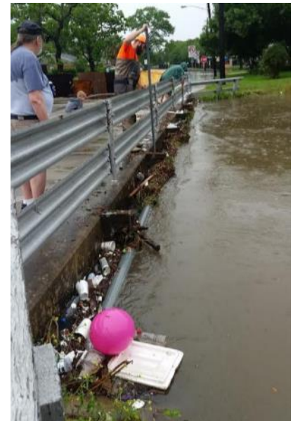
Residents clean debris clogged at the Landsdowne bridge over Willow Waterhole Bayou. Please keep your storm drains clear of debris.
