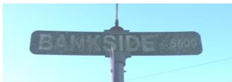
Street sign with grime and mold
