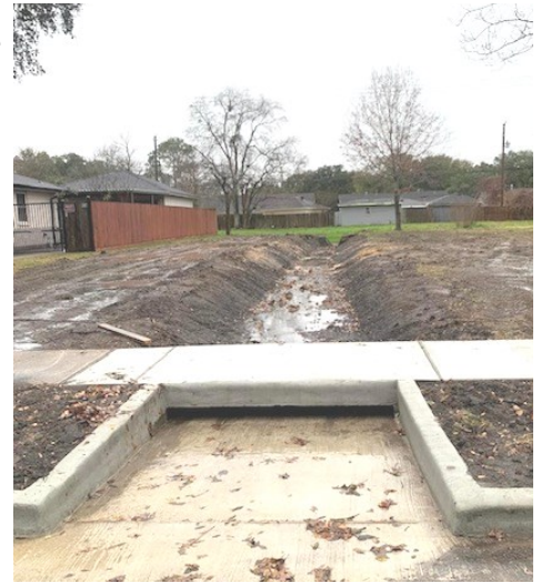
New drainage outlet on Beaudry
